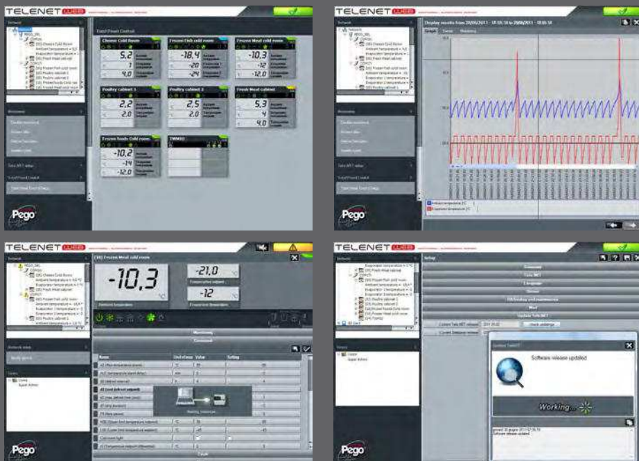
Screenshot demonstration of TeleNET monitoring system
