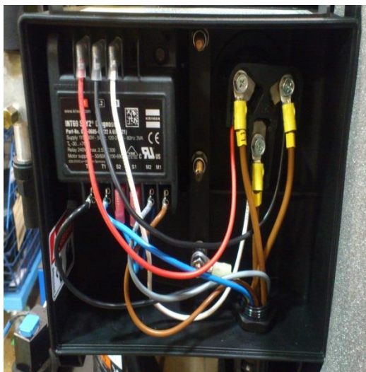
Figure 15: Correct electrical installation with cable glands for IP54 T-box (model ZF33KVE)
