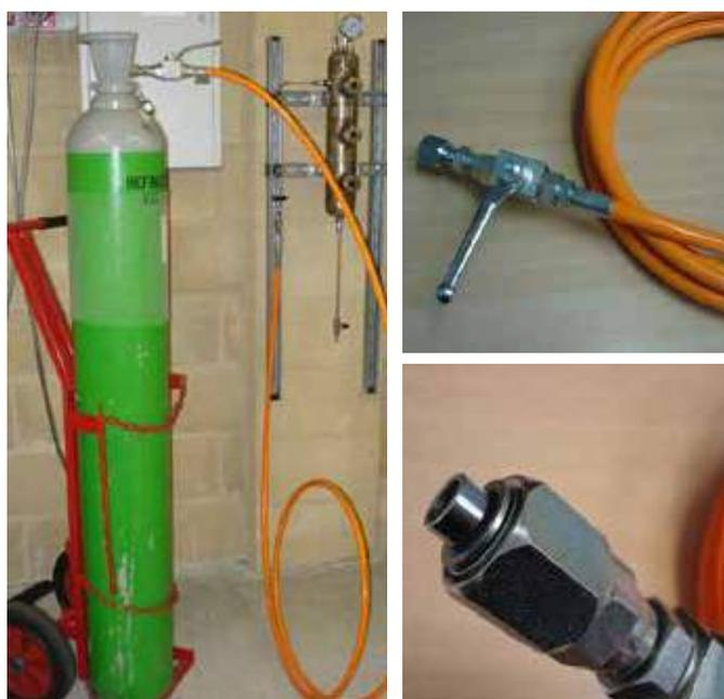
Figure 25. Example of R744 charging equipment
